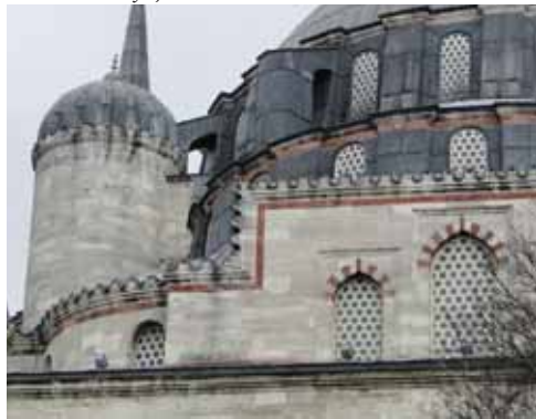
Fig. 20: Şehzade Mosque, a detail from the southwest façade
