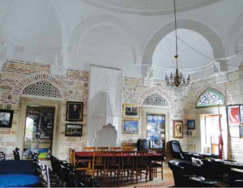
Fig. 101: Interior of the primary school classroom
