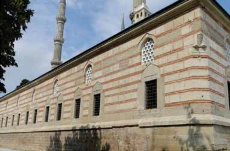
Fig. 98: Northeast corner and southeast façade of the Darulhadith
