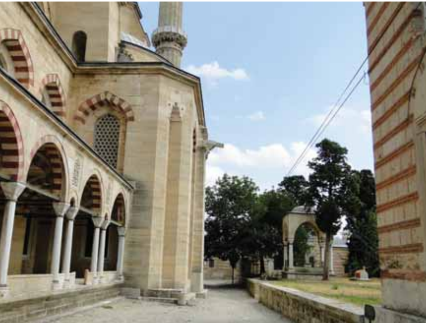
Fig. 86: Arcade in front of the qibla façade
