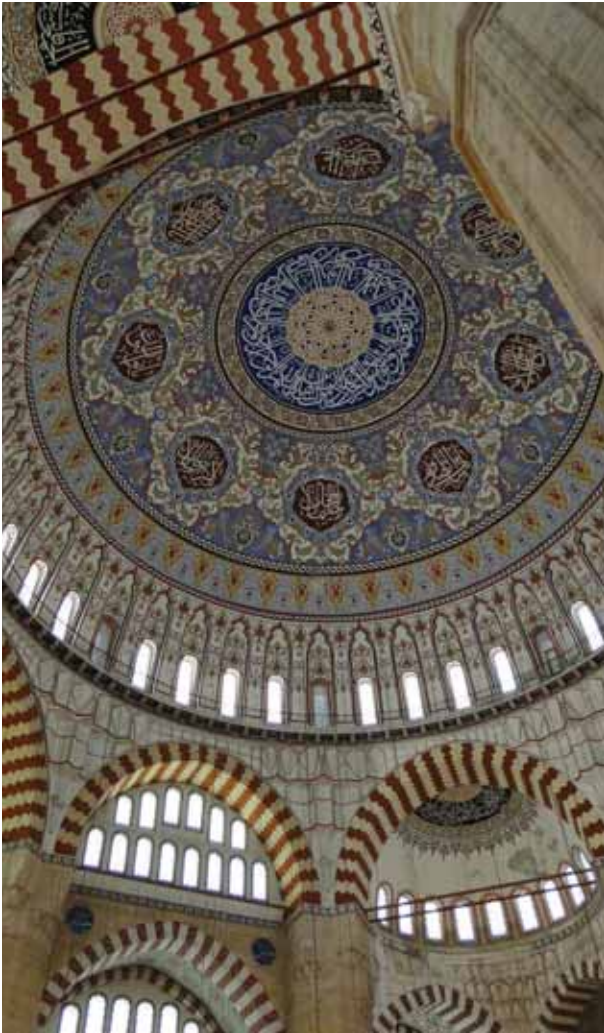
Fig. 78: Main dome suspended on eight arches
