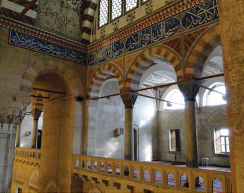
Fig. 65: Buttracing system and the women's gallery on the southwest wall
