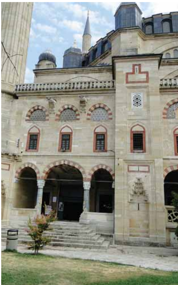
Fig. 80: Northwest elevation, side entrance to the mosque
