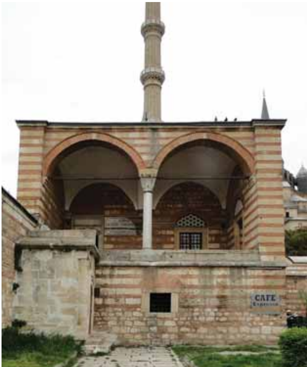
Fig. 99: Primary school, entrance façade
