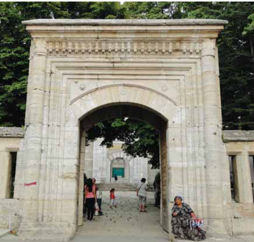
Fig. 27: Entrance to the enceinte from the northwest
