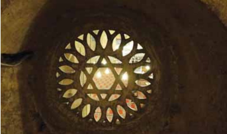
Fig. 64: Window opening on the stair leading to the gallery
