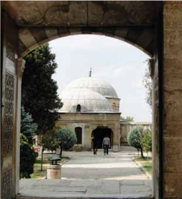
Fig. 32: Entrance to the enceinte from southwest; connection to the covered bazaar
