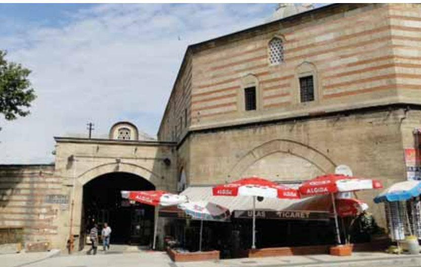
Fig. 93: Southeast corner of the darulKurra raised on vaulted shops next to the entrance of the covered bazaar
