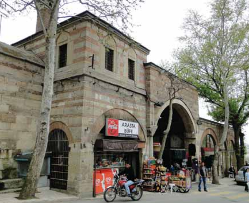
Fig. 104: Timekeepers room above the northwest entrance to the covered bazaar
