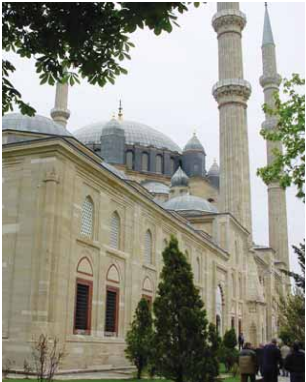
Fig. 36: Southwest wall of the courtyard and the corner with the attached column
